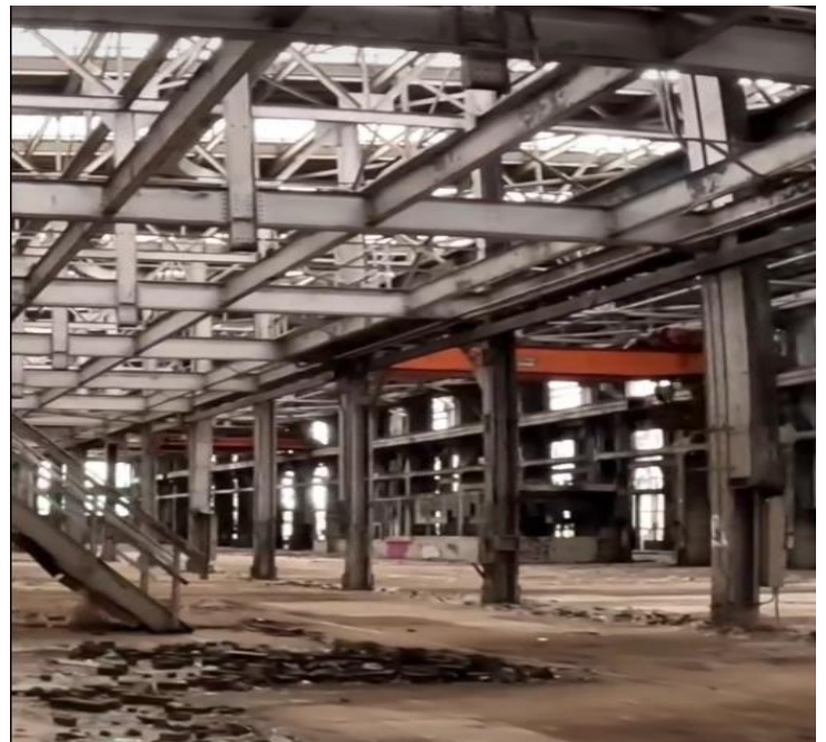
Former New Mexico ATSF Machine Shop
